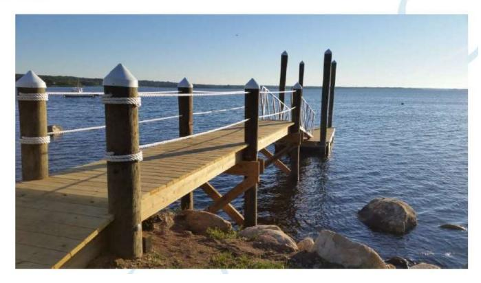
Thank you for the opportunity to present you with our proposal for the construction and installation of a residential boating facility consisting of a 4ft x 50ft fixed pier, a 3'x 16' ramp to a 8'x18'.75 float. (total length approximately 70') Based on a site visit as well as conversations this is a budgetary estimate and the project would consist of the following.
